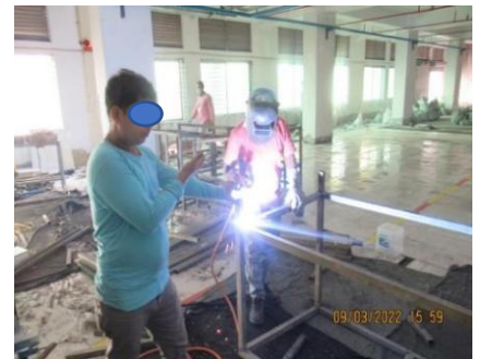
NC Picture 06: welding employees were not using hand gloves, mask, and helmet.
